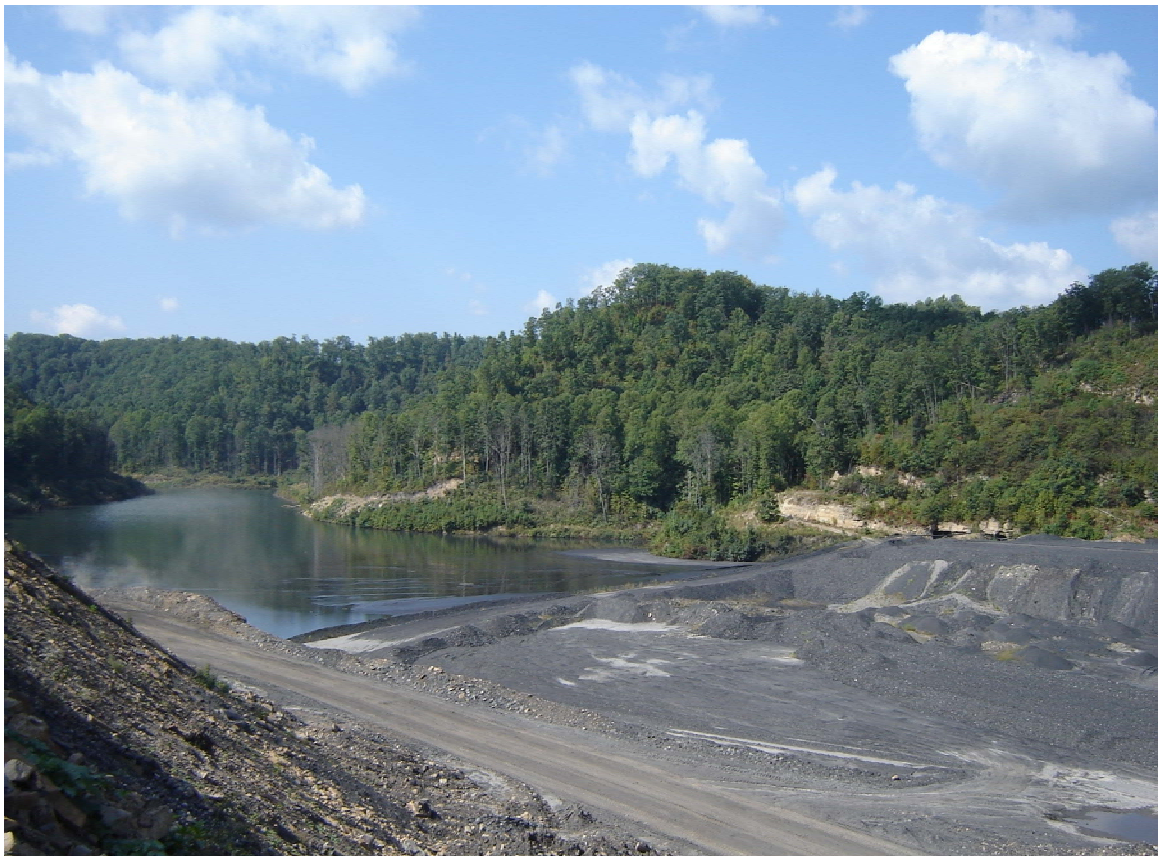
Lots Branch Tailings Impoundment
